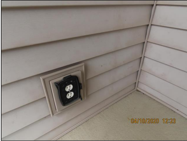
7.3 Item 1(Picture) front of home, near main entry
