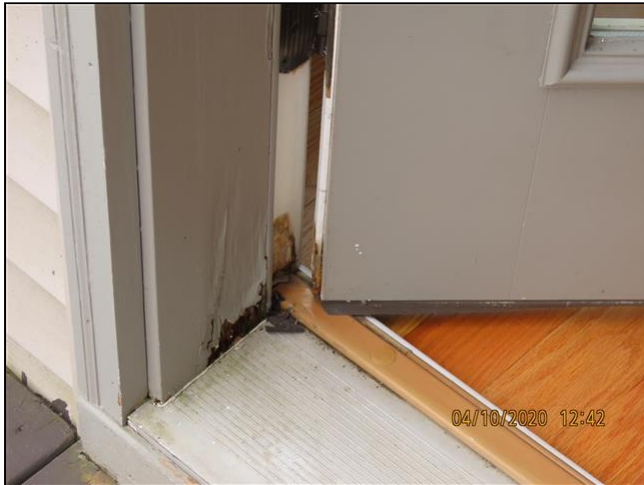
2.9 Item 1(Picture) rear of home, at deck
