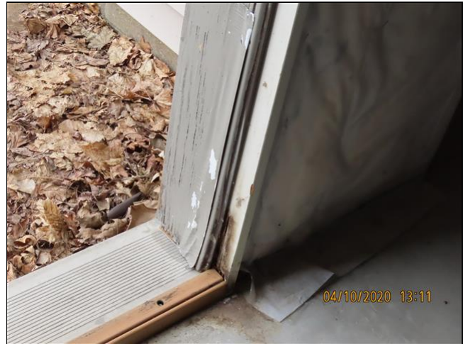
2.9 Item 2(Picture) rear of home, basement exterior door
