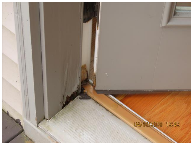
2.9 Item 1(Picture) rear of home, at deck
