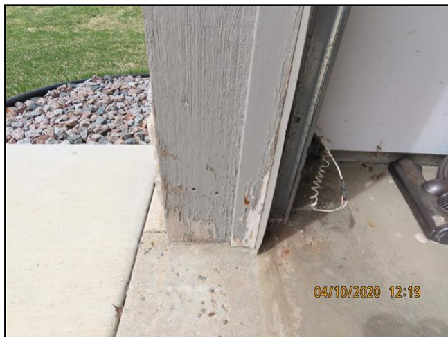
2.3 Item 2(Picture) garage door trim
