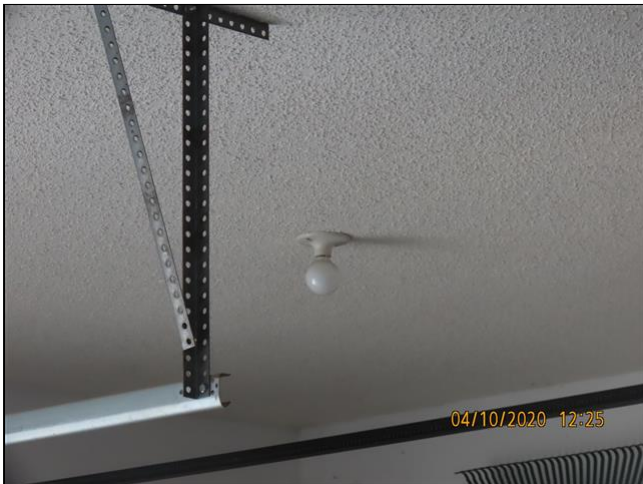
7.4 Item 1(Picture) garage
