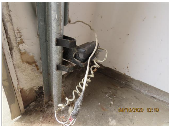
3.2 Item 1(Picture) localized moisture near overhead garage doors
