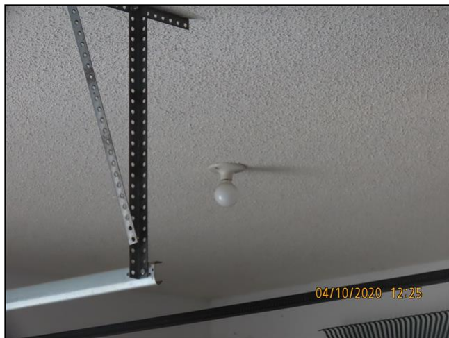
7.4 Item 1(Picture) garage
