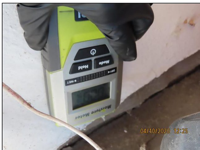
3.2 Item 3(Picture) area(s) dry at time of inspection.
